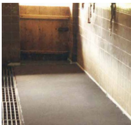
Couloir stabulation entravée p. 32
